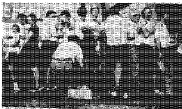
An informal static load test of a reject canard loaded at the Miami seminar. Sixteen men wrestle for room while Mike measures the butline of everyones feet! A non-catastrophic failure occurred near a hinge fitting at about 11.5 -g.
