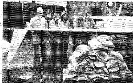
PETER KRAUSS AND HIS CREW OF HELPERS. IT TAKE A LOT OF MUSCLE TO LOAD SANDBAGS.
